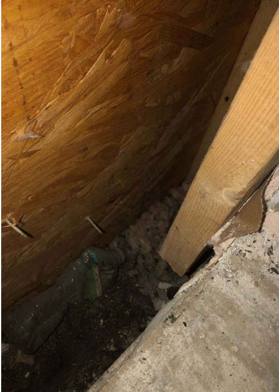
DAMAGED STUDS USED FOR REPAIRS ARE FLOATING ABOVE THE BASE - HAND SHOWS AIR SPACE UNDER THE BOTTOM OF STUD OSB SHEATHING USED FOR REPAIRS DETACHED FROM THE WALL STUD
