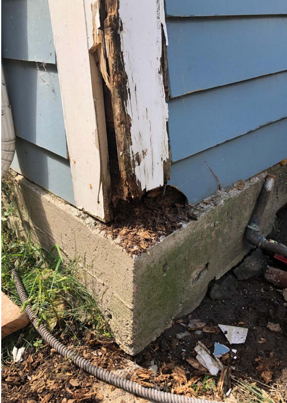
FULLY DAMAGED CORNER POST AND CONCRETE BASE FLOATING ABOVE THE GRADE
