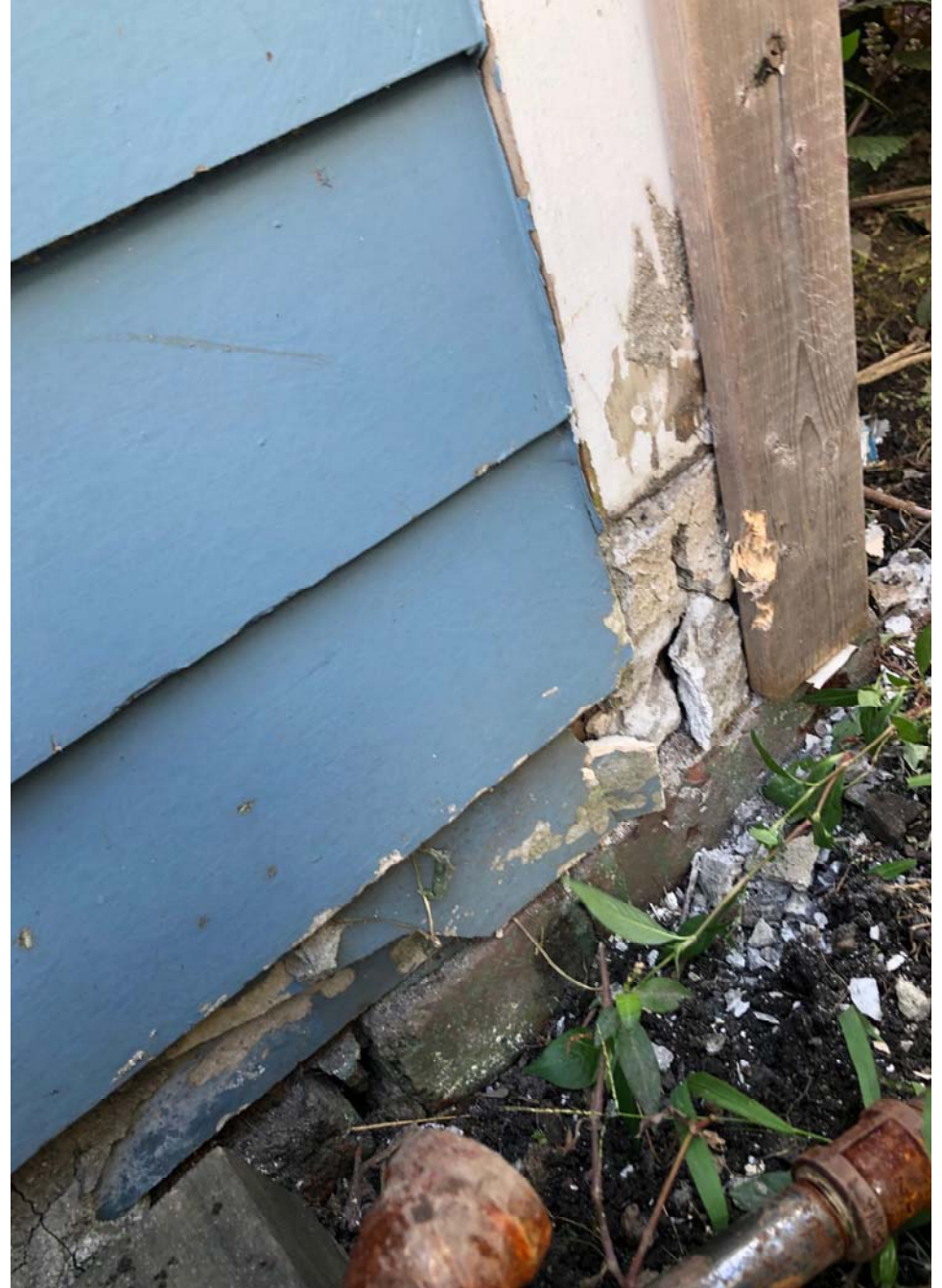
DAMAGED TO OTHER CORNER POST AT BASE AND DISINTEGRATED FOUNDATION TOP
