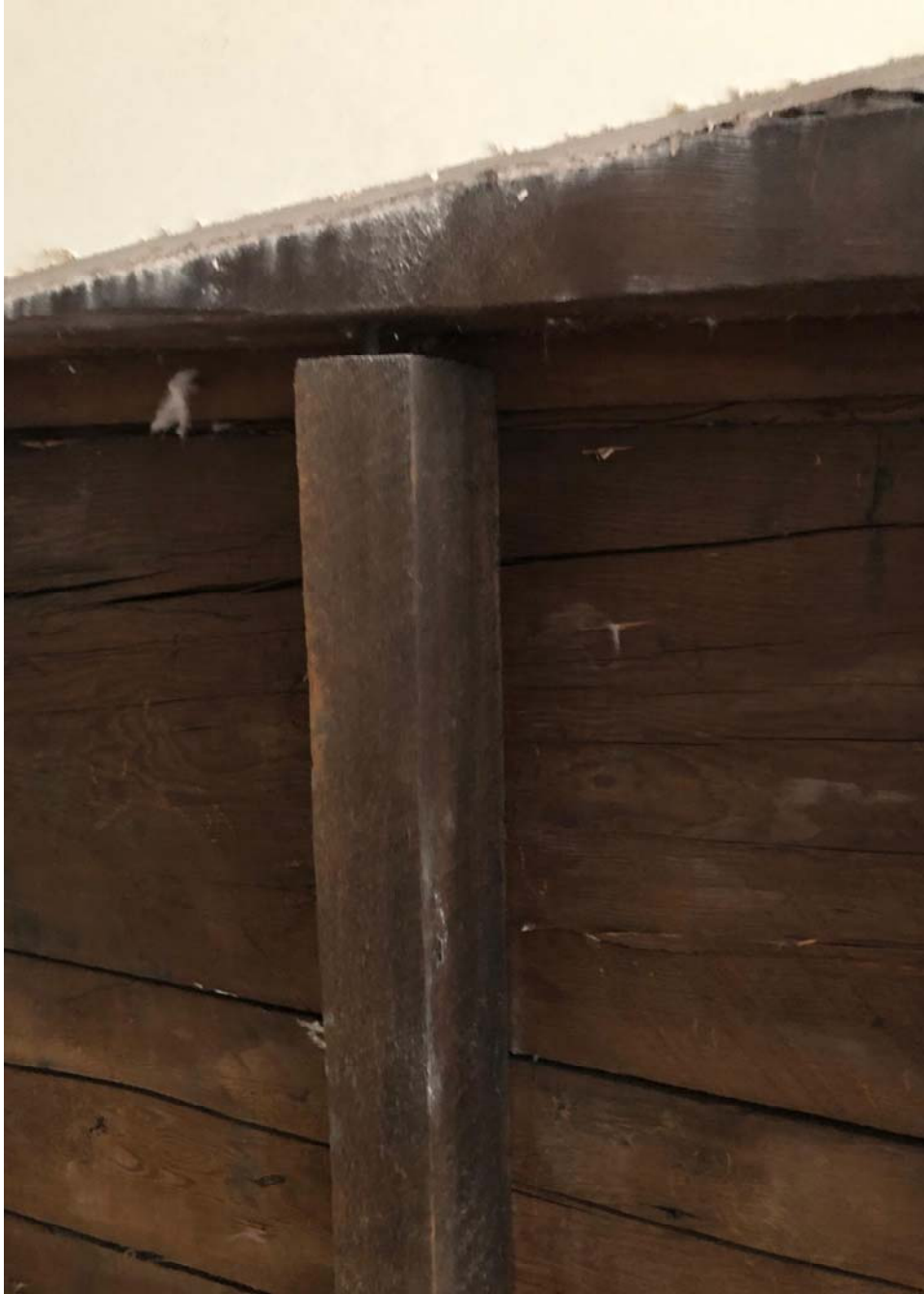
STUDS DETACHED FROM THE ROOF EAVE BEAM AND DRY ROT IN THE WALL SHEATHING BOARDS WITH SEVERAL CHECKS.
